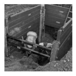
With telescoping spreaders and removed bottom panel
