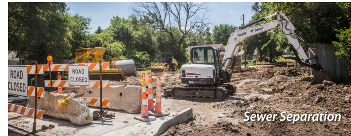
South Interceptor Force Main Tunnel Drilling
