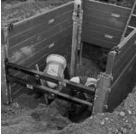
With telescoping spreaders and removed bottom panel
