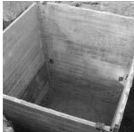
Stacked BUILD-A-BOX™ Modular Trench Shield System
