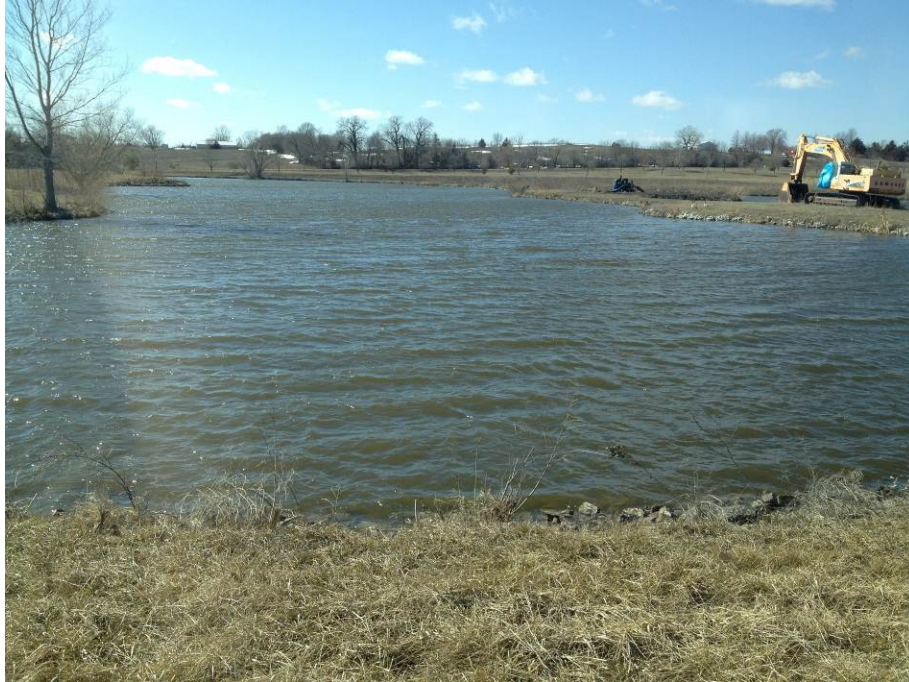
Photograph 1: View of SN-26 looking west, March 18, 2013.
