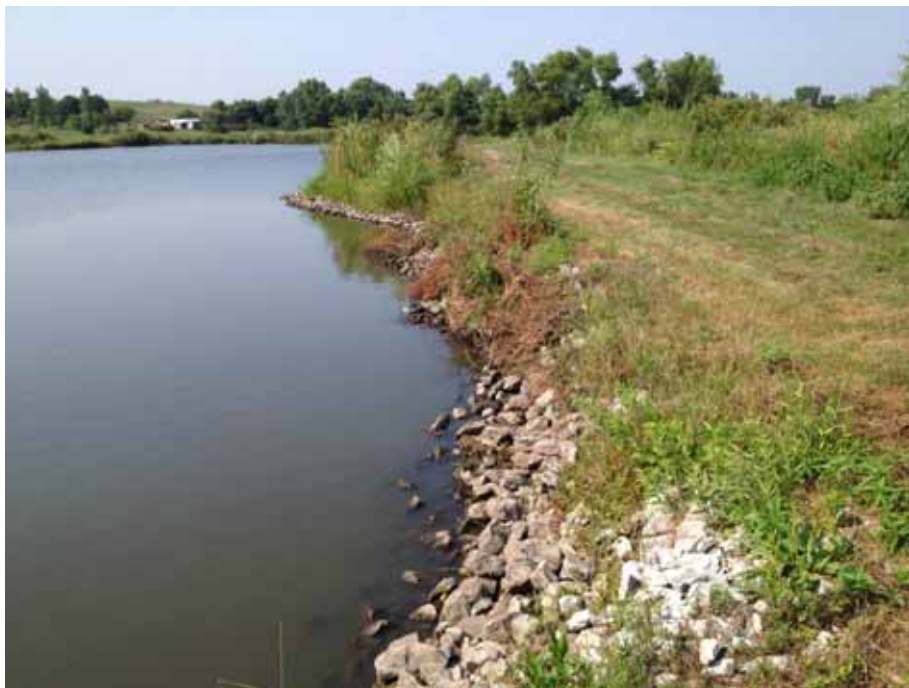
Photograph 4: View of SN-25 looking northwest, August 21, 2013
