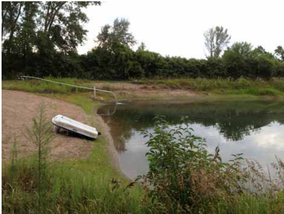
Photograph 8: View of DG-11 looking north, August 21, 2013.
