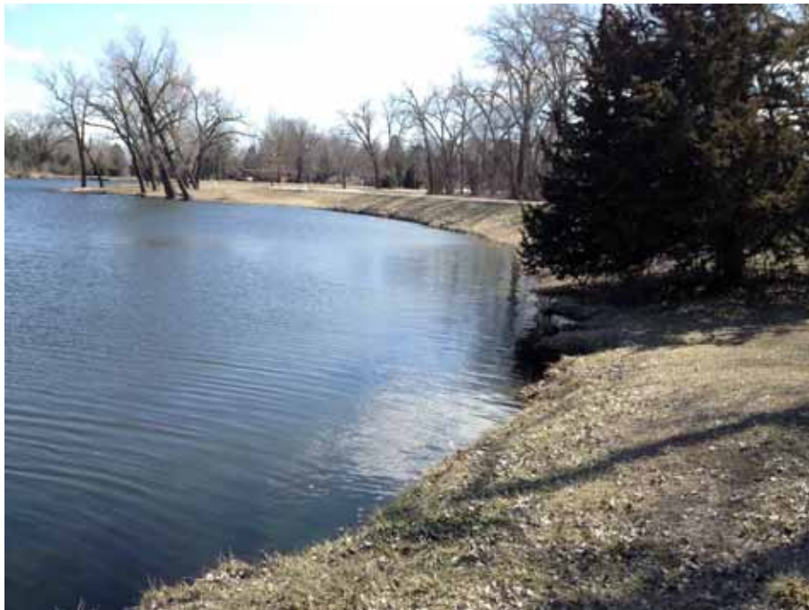
Photograph 2: View of DG-29 looking southeast, March 18, 2013.
