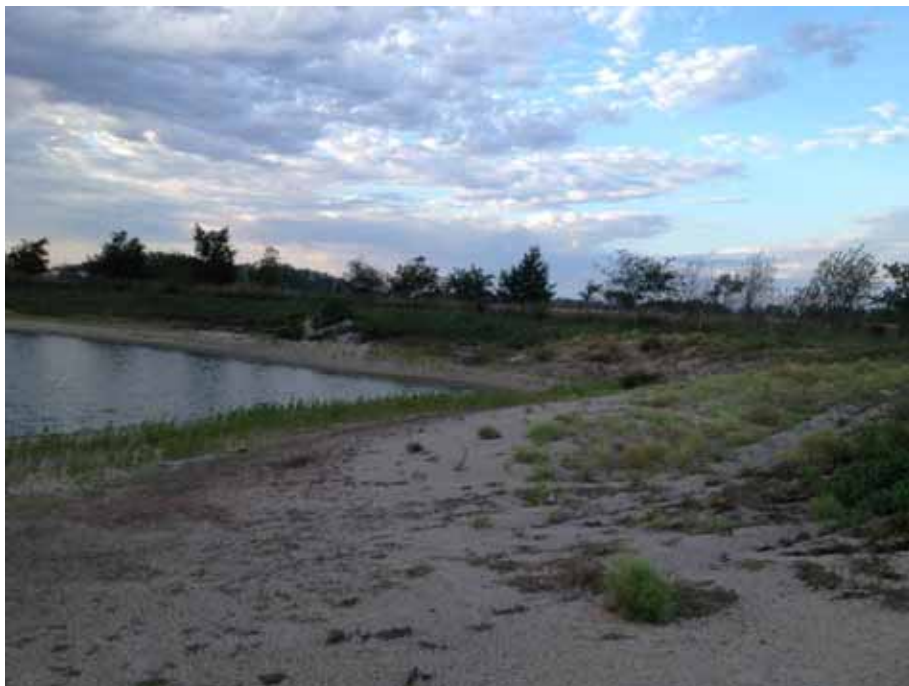
Photograph 8: View of DG-04B looking southwest, September 26, 2013.
