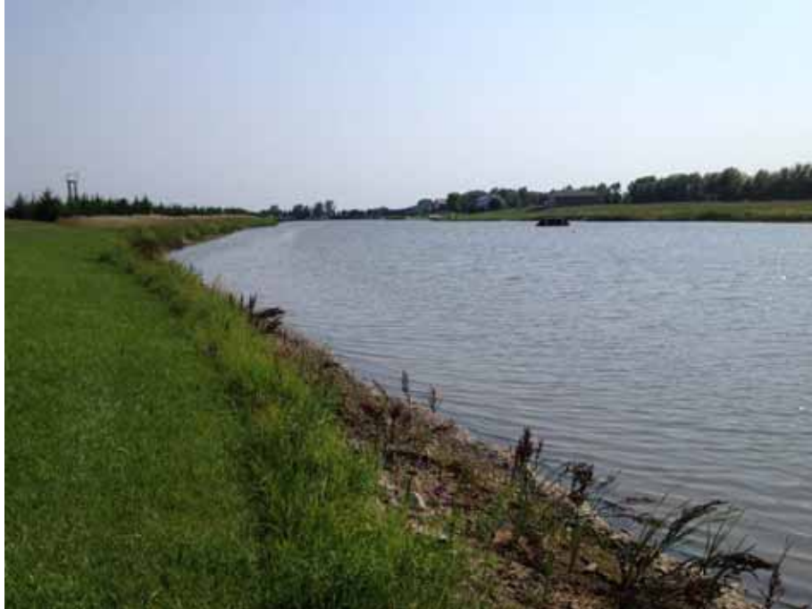
Photograph 3: View of SN-27 looking south, August 21, 2013.
