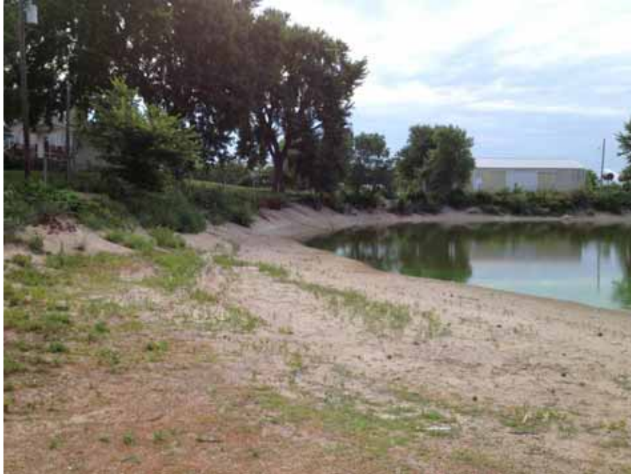
Photograph 3: View of DG-04B looking southeast, August 21, 2013.
