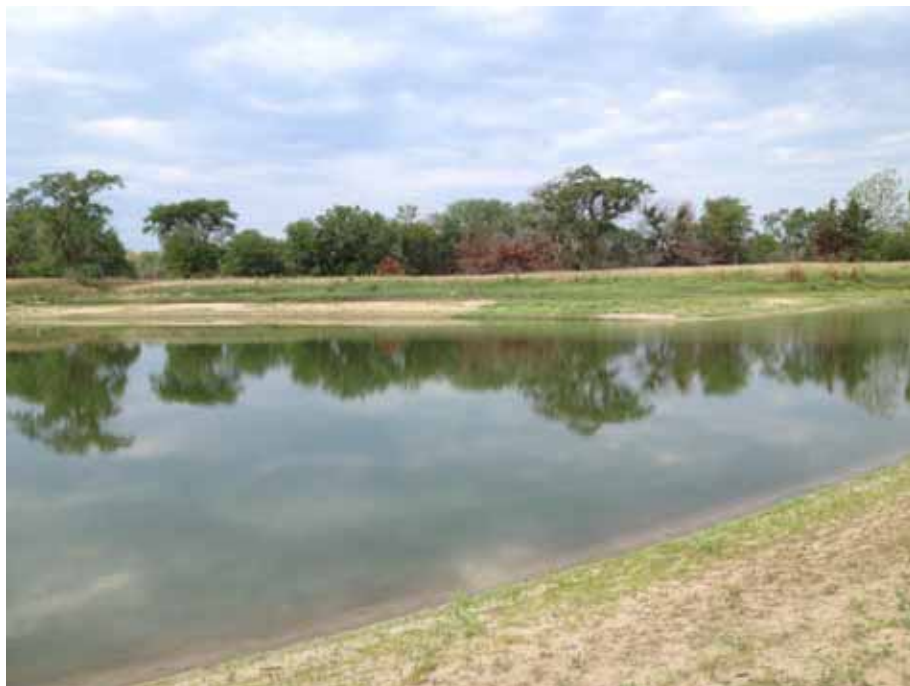
Photograph 4: View of DG-52 looking west, August 21, 2013.
