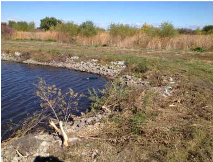
Photograph 8: View of SN-25 looking northwest, October 24, 2013.
