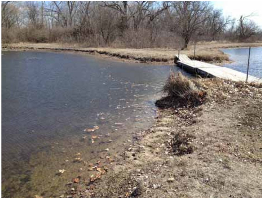
Photograph 2: View of DG-30 looking southeast, March 18, 2013.
