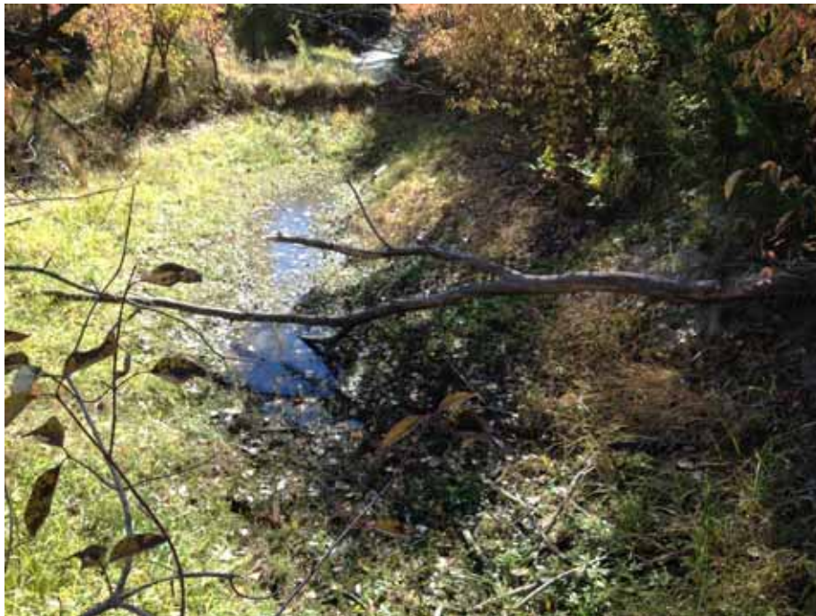
Photograph 4: View of DG-20D looking southeast, October 24, 2013.
