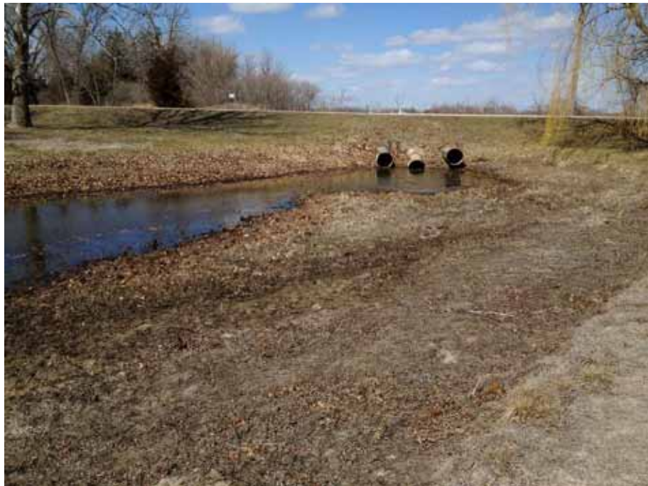
Photograph 2: View of DG-32 looking northwest, March 18, 2013.
