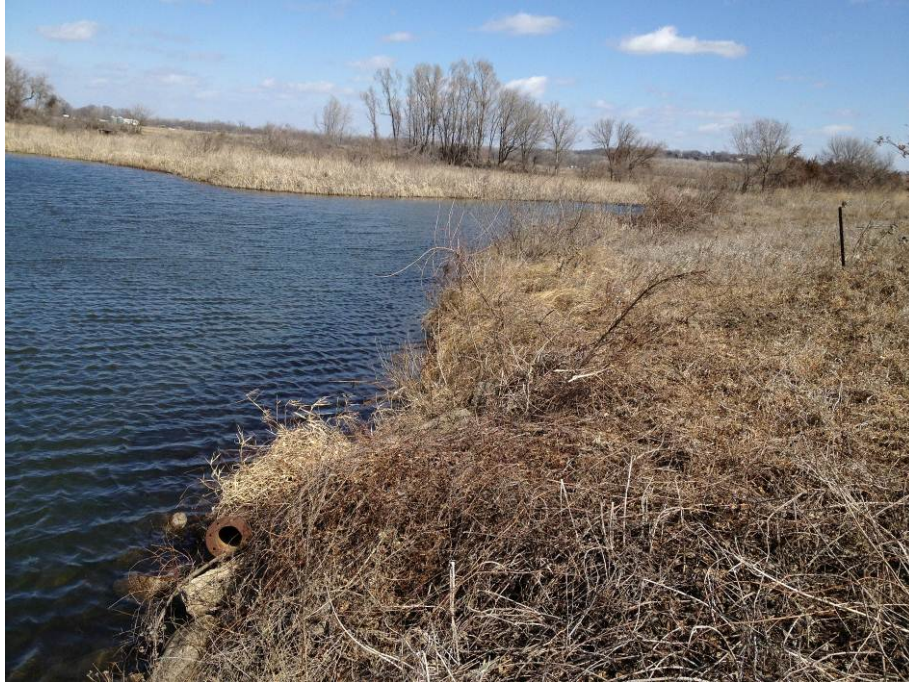
Photograph 3: View of DG-03 looking east, March 18, 2013.
