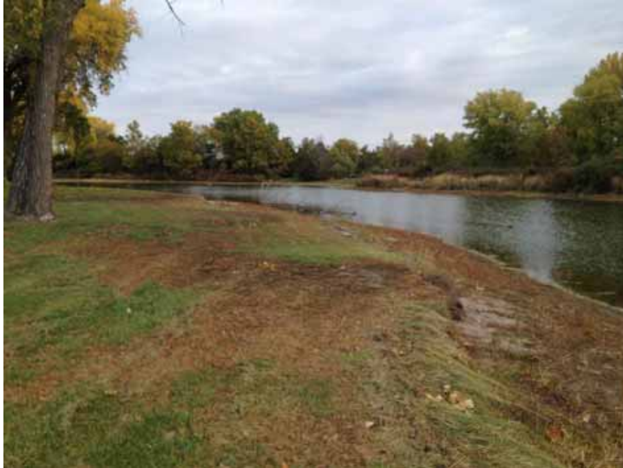
Photograph 7: View of DG-30 looking north, October 25, 2013.
