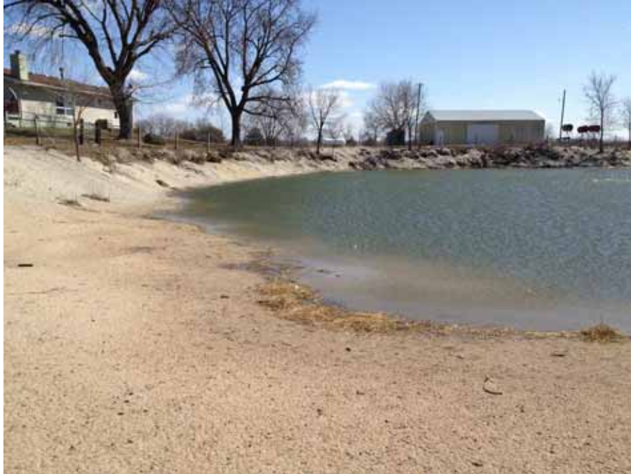
Photograph 1: View of DG-04B looking southeast, March 18, 2013.
