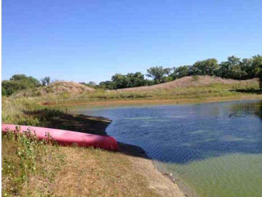
Photograph 5: View of DG-23A looking northeast, September 26, 2013.
