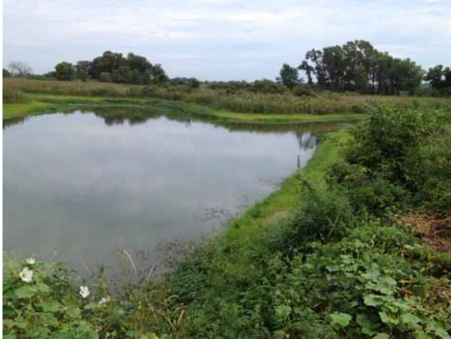
Photograph 7: View of DG-03 looking east, August 21, 2013.
