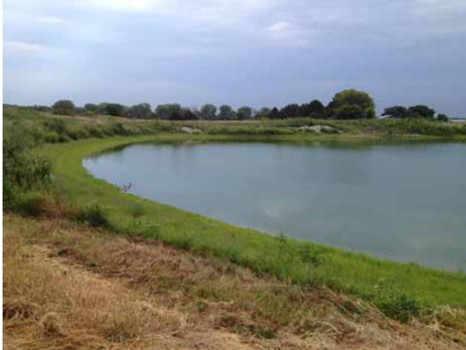
Photograph 3: View of DG-01 looking east, August 21, 2013.
