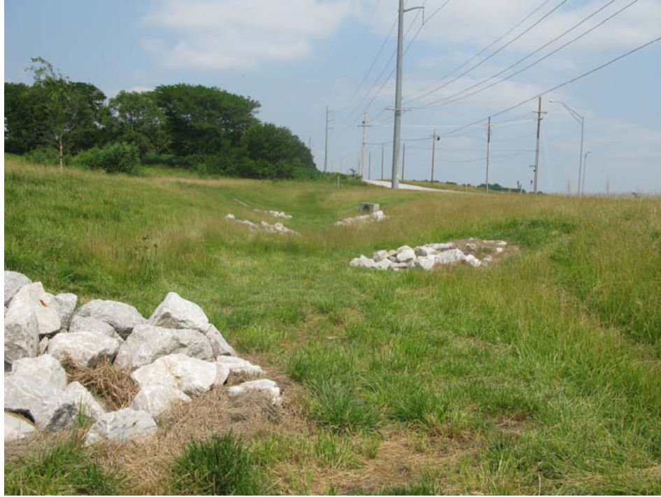
Photo 1: View east of the Stream Mitigation Site (June 2012).
